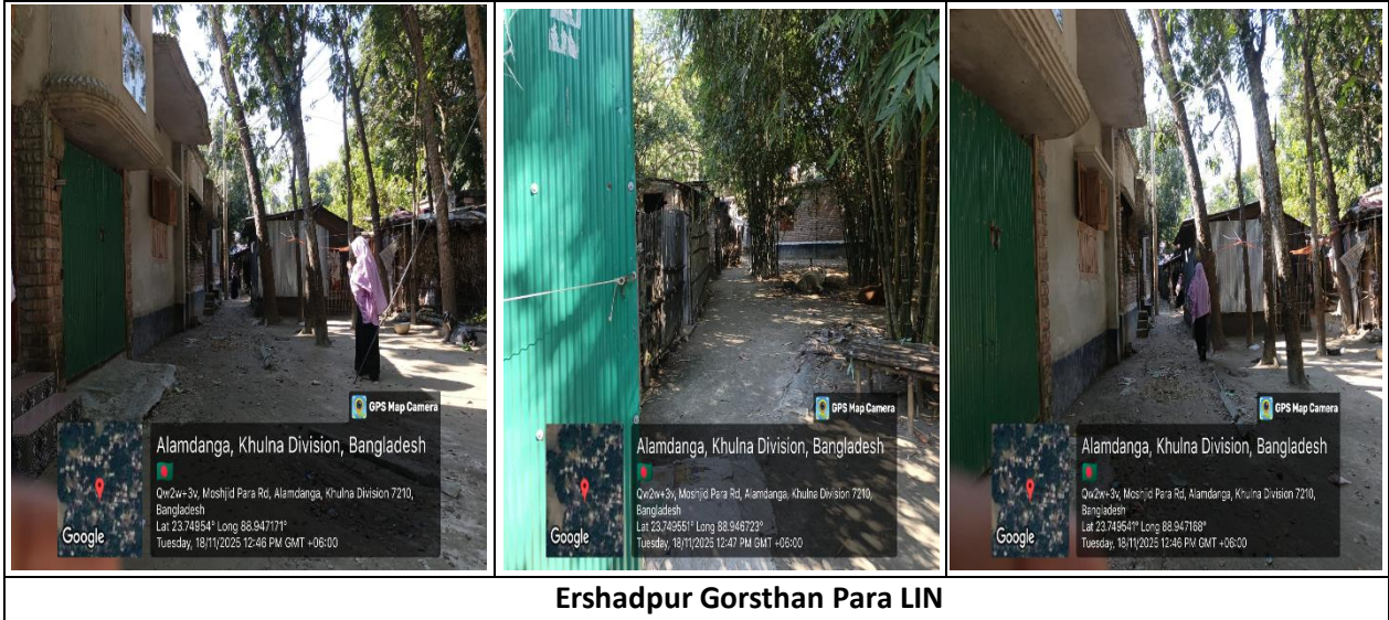
• Figure IV.7: Existing Situation at Ershadpur Gorsthan Para LIN
