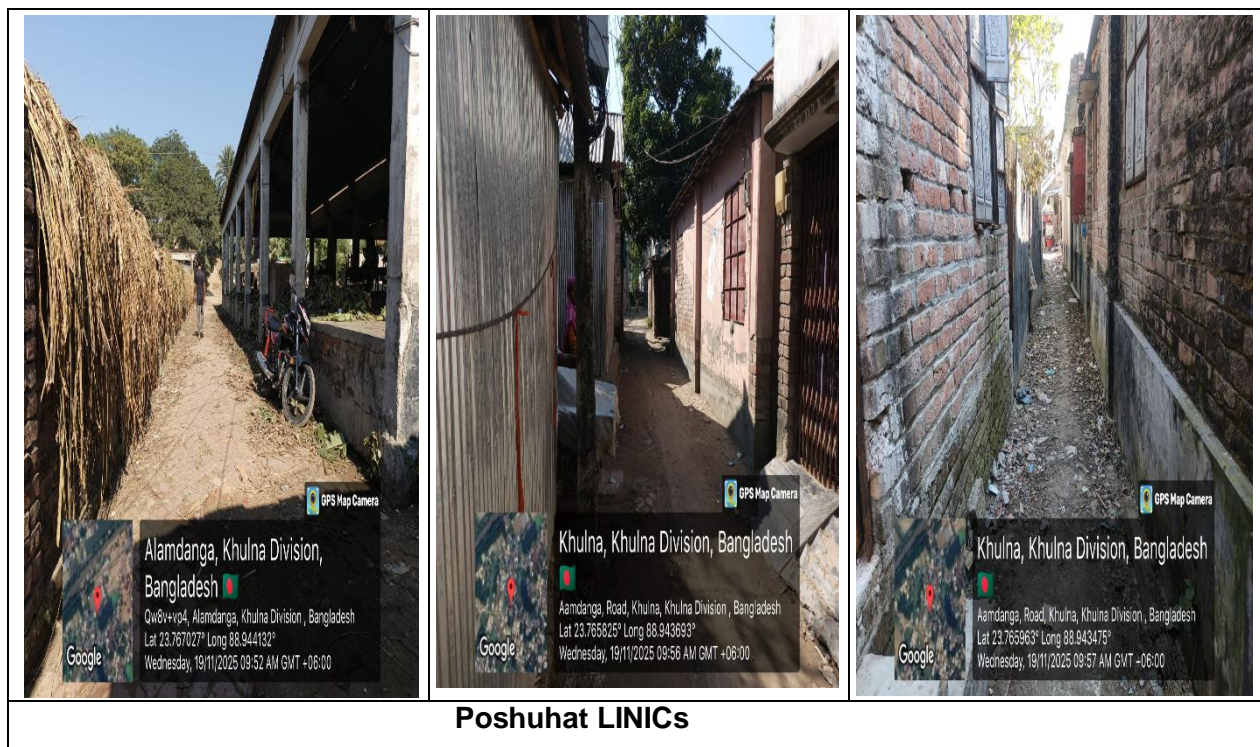
Figure IV.4: Existing Situation at Posuhat LIN
